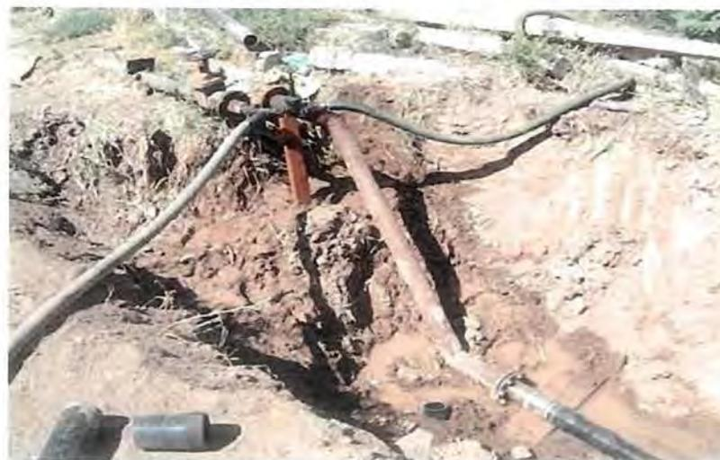
Figure D-18 (U): Connection with New Water Line in Operations Area
